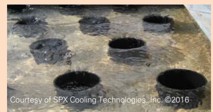
Figure 2. Marley VariFlow™ Nozzle Cap
