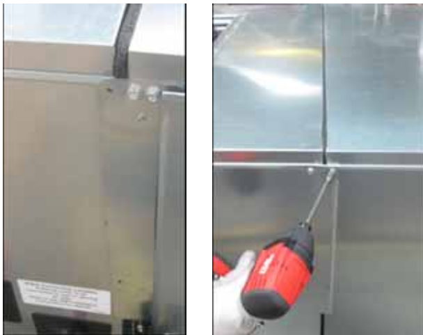
Figure 27. Bring sections together, align holes.
