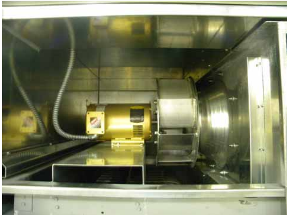
Figure 68. Indoor fan and motor
