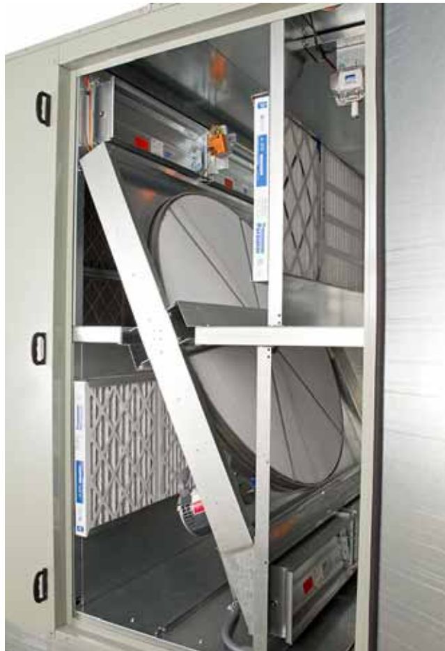
Figure 67. Total-energy wheel module
